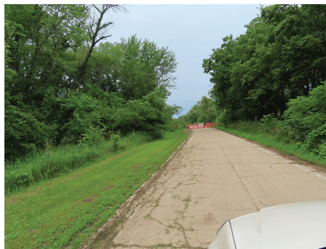
Existing photo 3c: Photo taken from Lincoln Highway Heritage Byway looking westerly towards what is known as the overflow bridge. The overflow bridge is being replaced and will be opened to vehicular access, but the Wapsi bridge, which is located farther west and is closed as well, will not be open for vehicular traffic.
