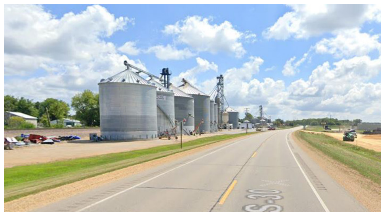
Existing photo 8a: Photo taken entering the west side of Wheatland via Hwy. 30
