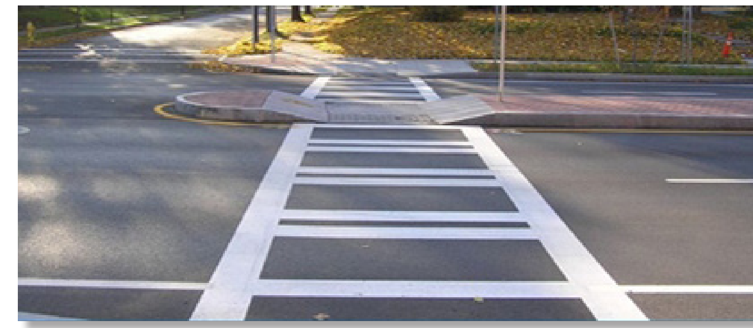
Figure B: Raised median with crosswalk cut-through (aka refuge island); Photo source: highways.dot.gov
