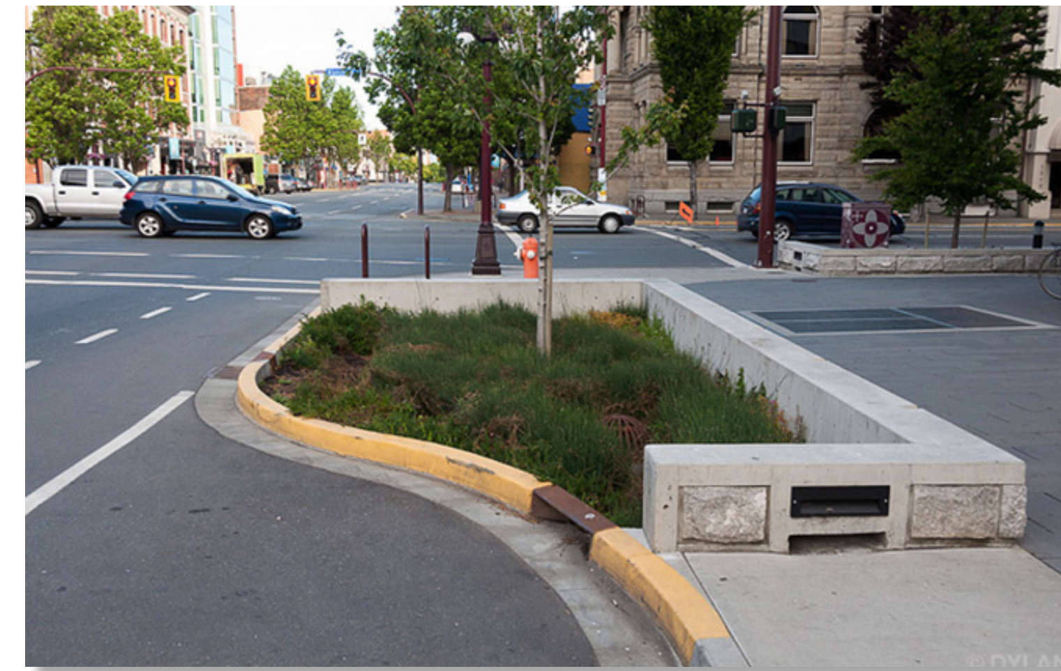
Figure C: Curb Extension (also referred to as bulb-out or bump-out); Photo credit: Dylan Passmore
