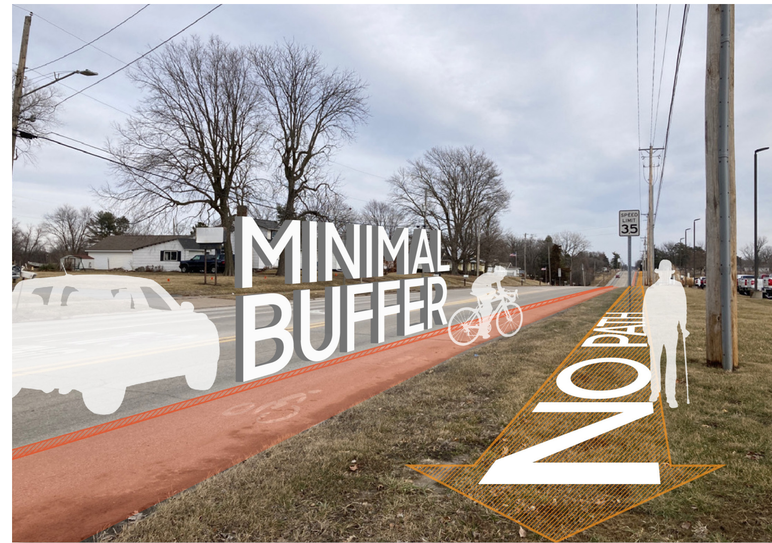
Mt. Pleasant Street is intimidating to both cyclists and pedestrians because the bike lane is too close to vehicular traffic and there is no sidewalk or trail.
