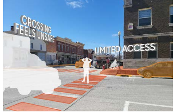
Accessibility and safety are issues when crossing at Downey and Main Street due to faded crosswalks, no ramps, and aging infrastructure.
