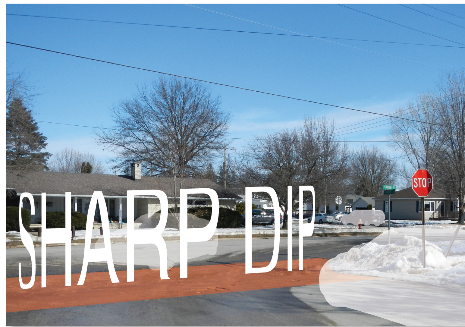
The dip in the road at East 4th and Monroe Streets can damage cars and contributes to poor drainage.
