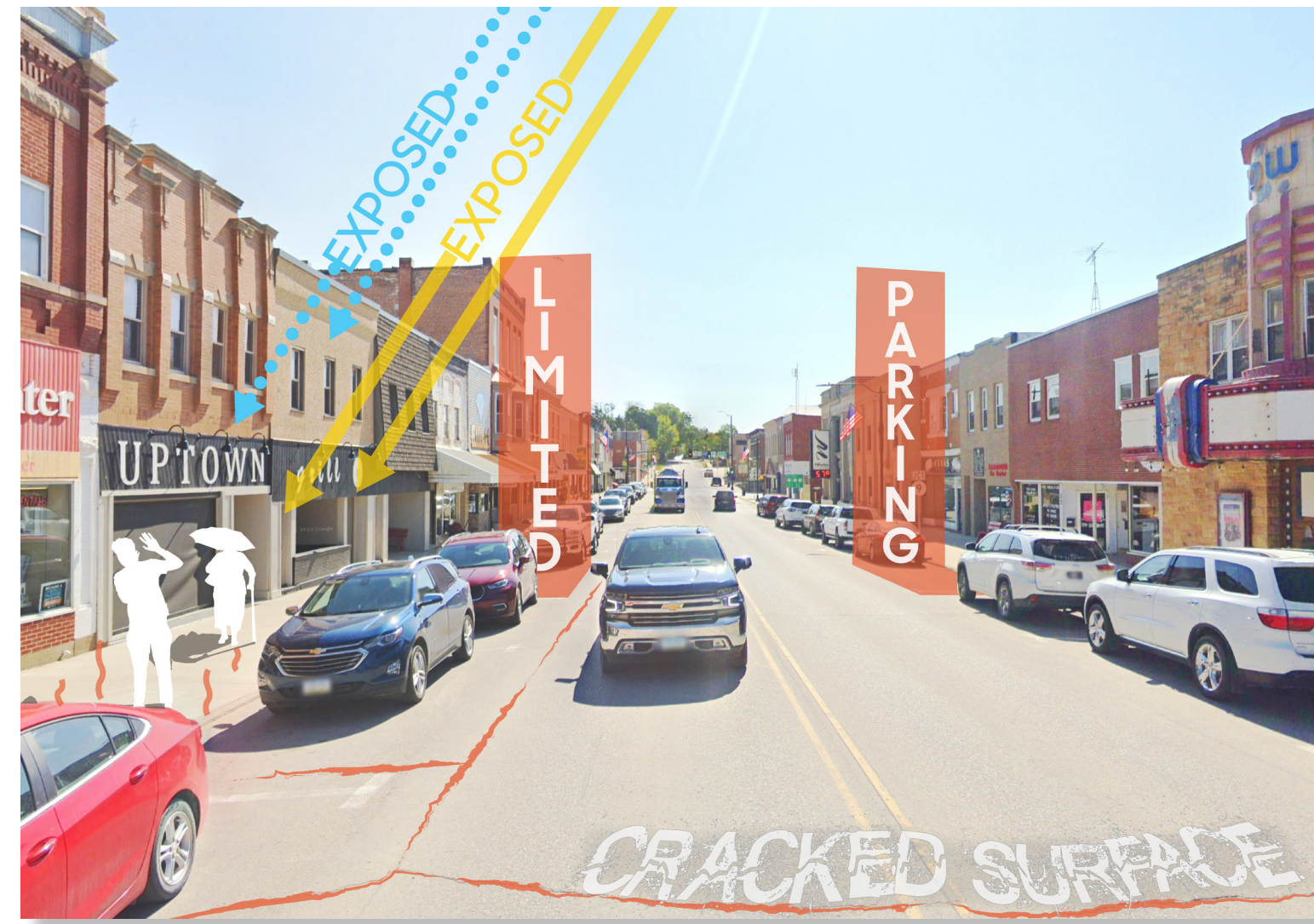
Waukon's Downtown has limited protection from the elements, and the street is cracked and has insufficient parking to accommodate the heavy traffic.
