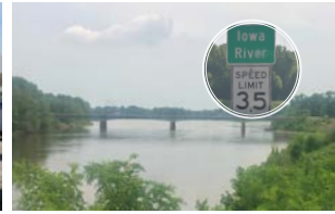
Existing Hwy 99 bridge Speed limit on Hwy 99 and 61
