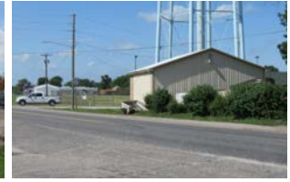
Existing crossing on Hwy 61
