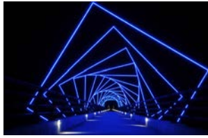
Light up bridge over Des Moines River, IA
