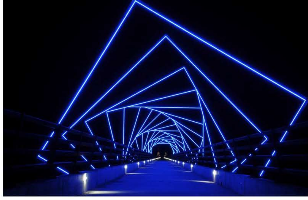
Light up bridge over Des Moines River, IA
