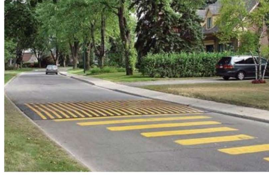
Raised speed bump crosswalk City of Lynchburg, VA
