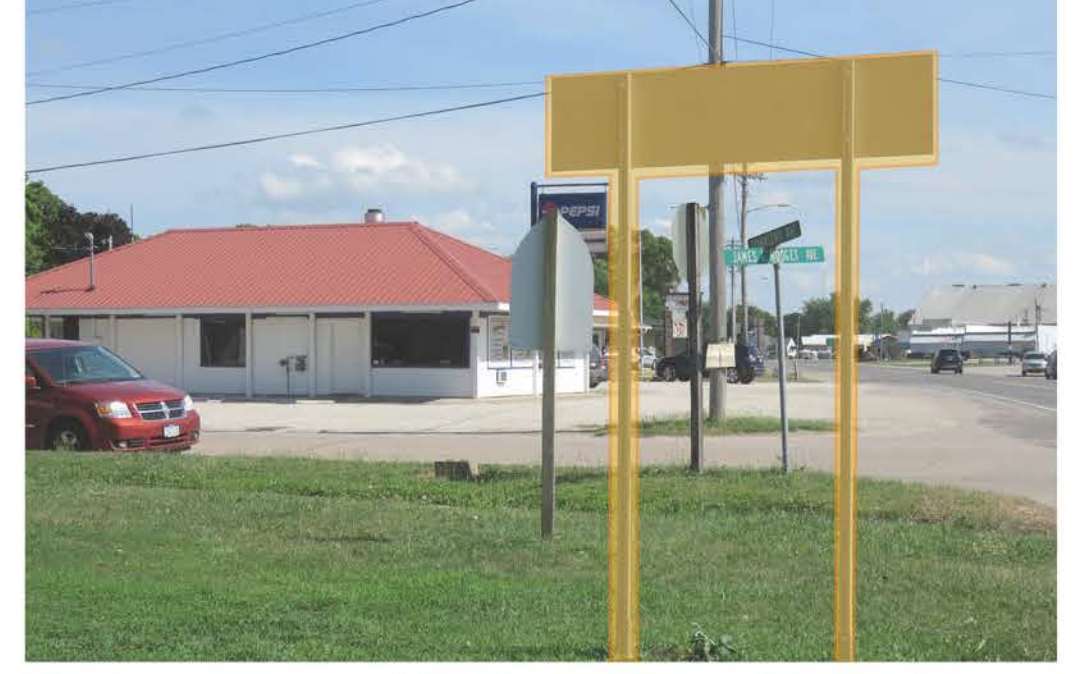
Reduce speed limit on Hwy 61 and replace signage to help visibility
