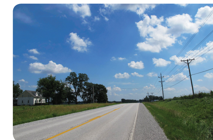
Existing 60th Avenue/Y40 corridor looking south toward Hwy. 6
