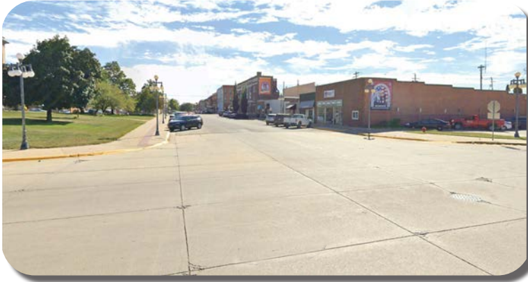
Photo of existing intersection from north side looking south along 1st Ave.
