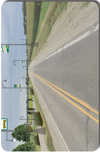
Separated 10-foot-wide trail bike trail: Hwy. 218 proposed enhancements (option 2, preferred/final)
