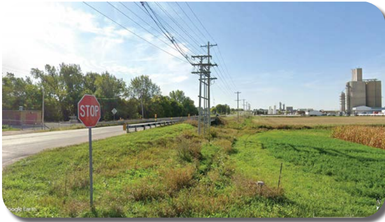
Existing Hwy. 218 (K Ave.) at Hinkle Creek - photo taken from north side of Hinkle Creek at intersection of 5th Street W. and Hwy. 218 looking southerly along Hwy. 218 toward Hinkle Creek
