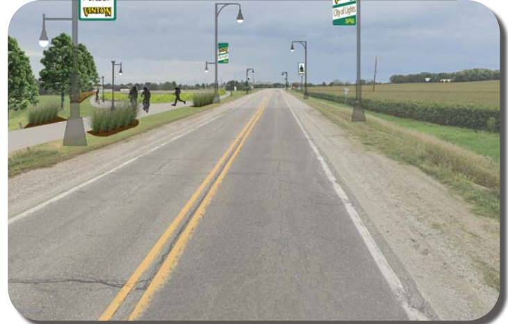
Separated 10-foot wide trail: Hwy. 218 proposed enhancements
