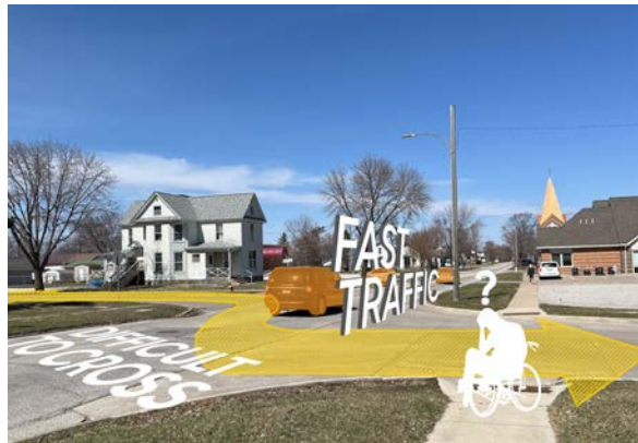
The confusing geometry and fast traffic at the intersection of 13th St. and C Ave. creates challenging crossing conditions for pedestrians.
