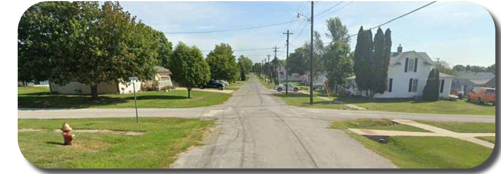
Incomplete sidewalk segments, sidewalks in ill-repair, and lack of ADA accessibility prevent safe pedestrian circulation.
