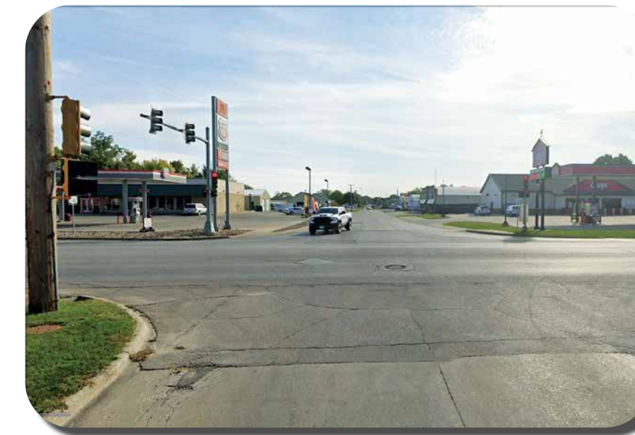
Existing Hwy. 218 & 4th St. intersection - photo taken from west side of Hwy. 218 looking easterly along 4th St.
