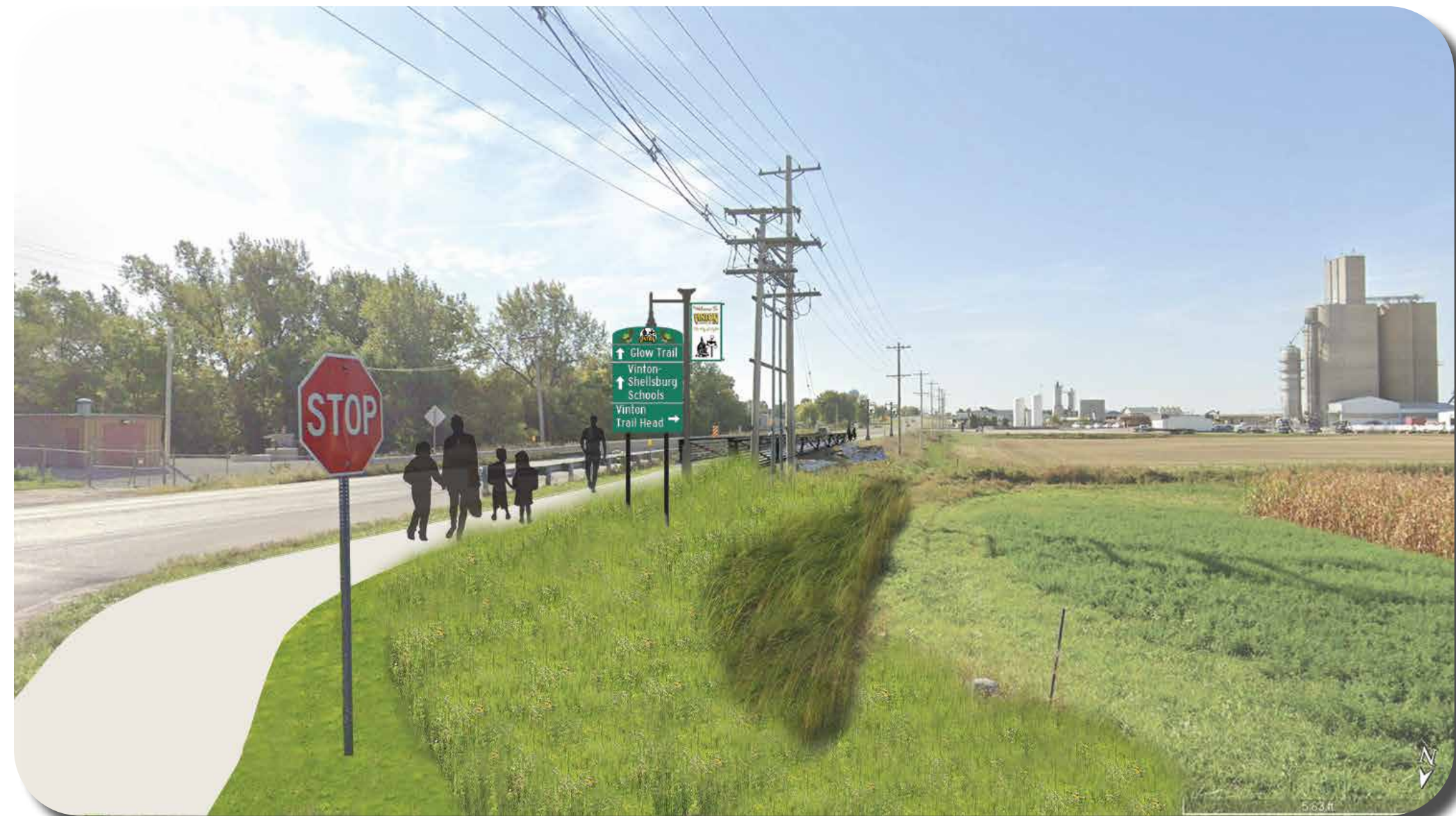
Proposed concept illustrates the following enhancements: 6-foot-wide ADA-compliant sidewalk, prefabricated pedestrian bridge, branded way-finding signage, decorative pedestrian lighting with banners, right-of-way planted with native prairie grasses and forbs, with wet ditch areas planted with appropriate native wet prairie/wetland vegetation such as prairie cord grass.
