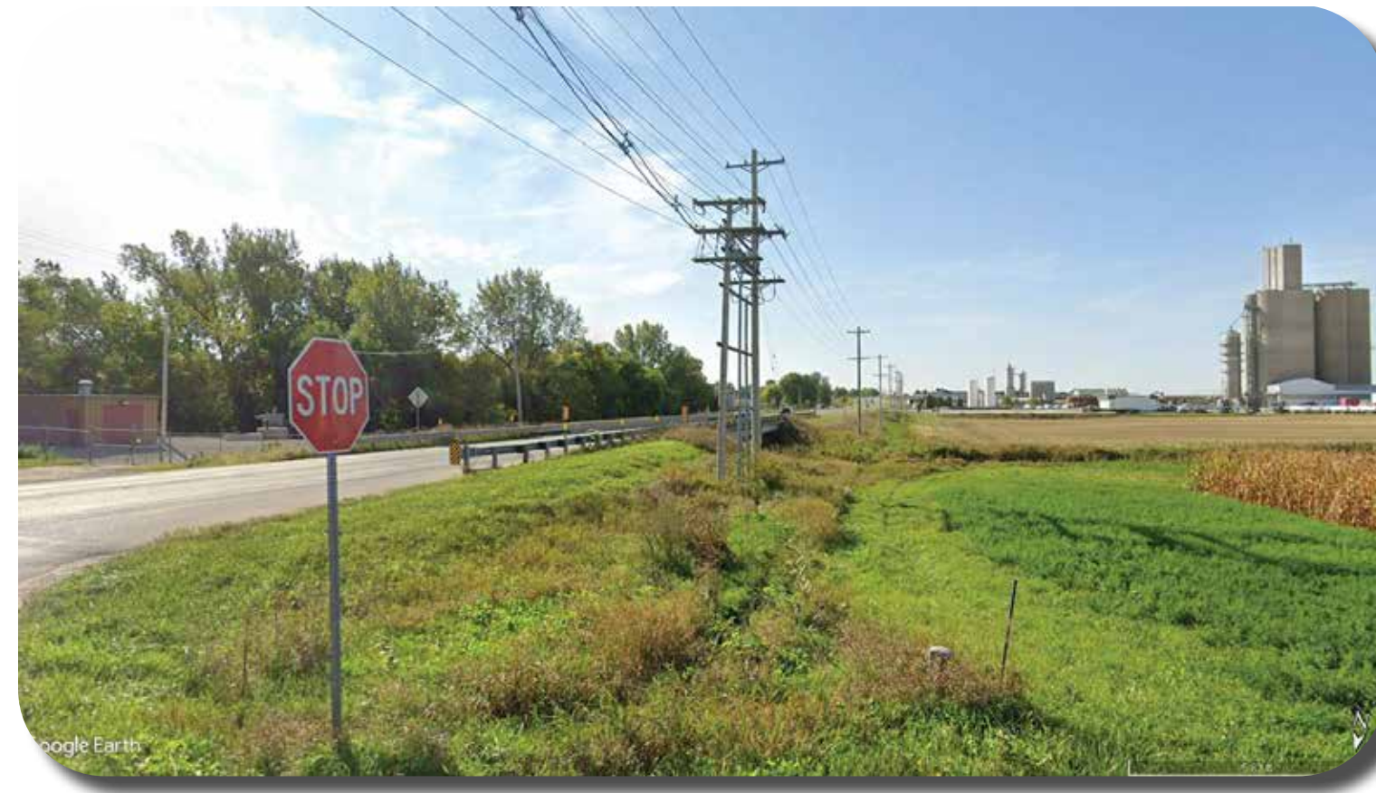
Existing Hwy. 218 (K Ave.) at Hinkle Creek - photo taken from north side of Hinkle Creek at intersection of 5th Street W. and Hwy. 218 looking southerly along Hwy. 218 toward Hinkle Creek
