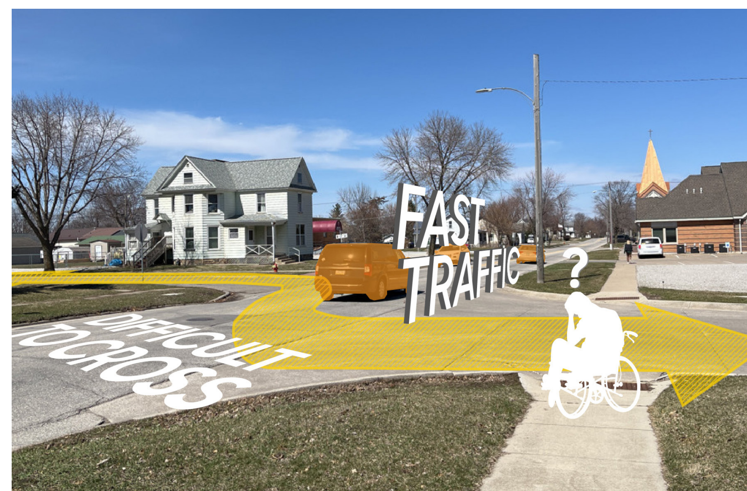
The confusing geometry and fast traffic at the intersection of 13th St. and C Ave. creates challenging crossing conditions for pedestrians.
