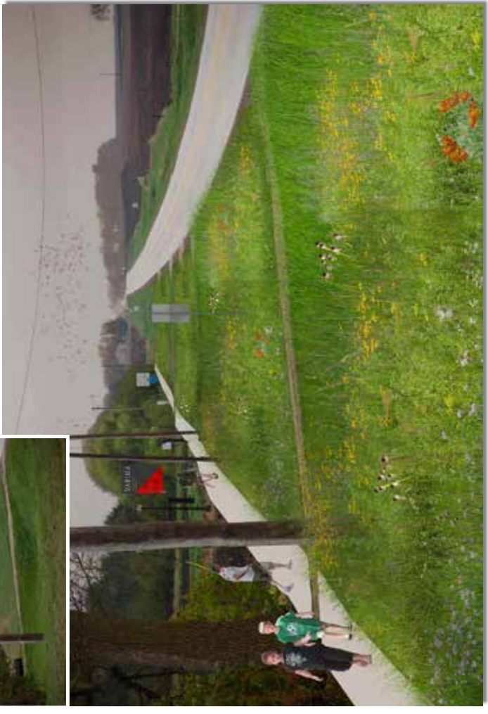
Before And After - Looking west on C49, added trail and prairie plantings within the ditch for beautification and stormwater management.
