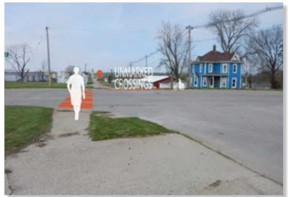
There is no marked or safe crossing across Broadway Street and US Business 30.
