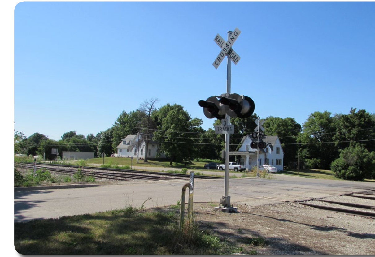
Railroad Intersection at South Western Avenue
