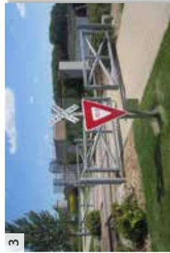
The safety of pedestrians and bicyclists crossing the railroad tracks can be improved by adding signage, barriers and level pavement transitions. An example of this from Waterloo, Iowa is also shown.
