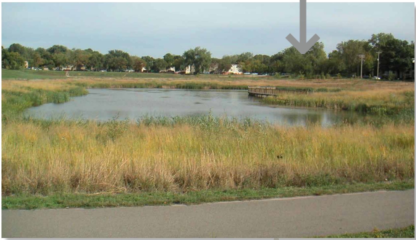
Creating a detention pond would allow for the run-off to be stored on-site and discourage excess water from flowing into the community
