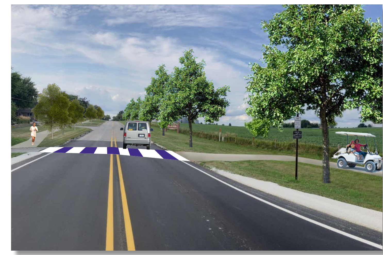
A side path trail in the eastern right of way of Linn Street crosses Linn Street at 10th Avenue to connect with a widened sidewalk. This expanded trail connects south of Highway 210 neighborhoods and Slater Cemetery visitors to downtown and the school. Roadside trees help to calm traffic and reduce wind.
