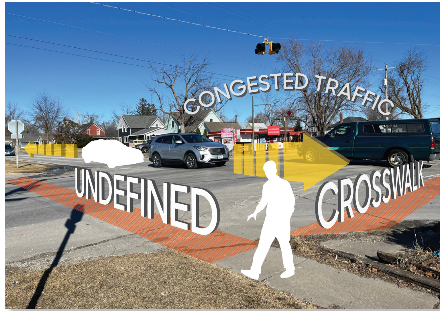
The crosswalks at Highway 210 and Linn Street are not well defined, and the four-way stop creates traffic congestion.
