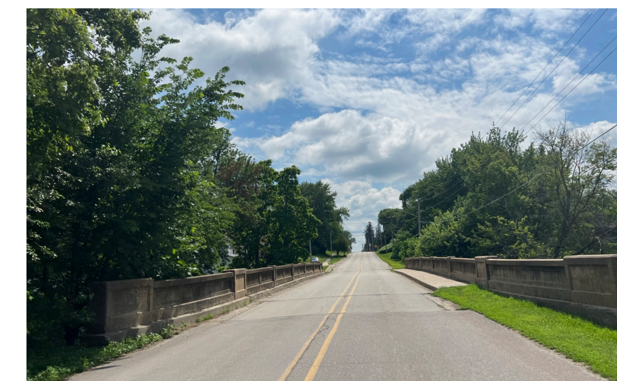
(C) South Cherry Street bridge
