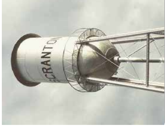
Scranton's water tower is the oldest working water tower in Iowa.
