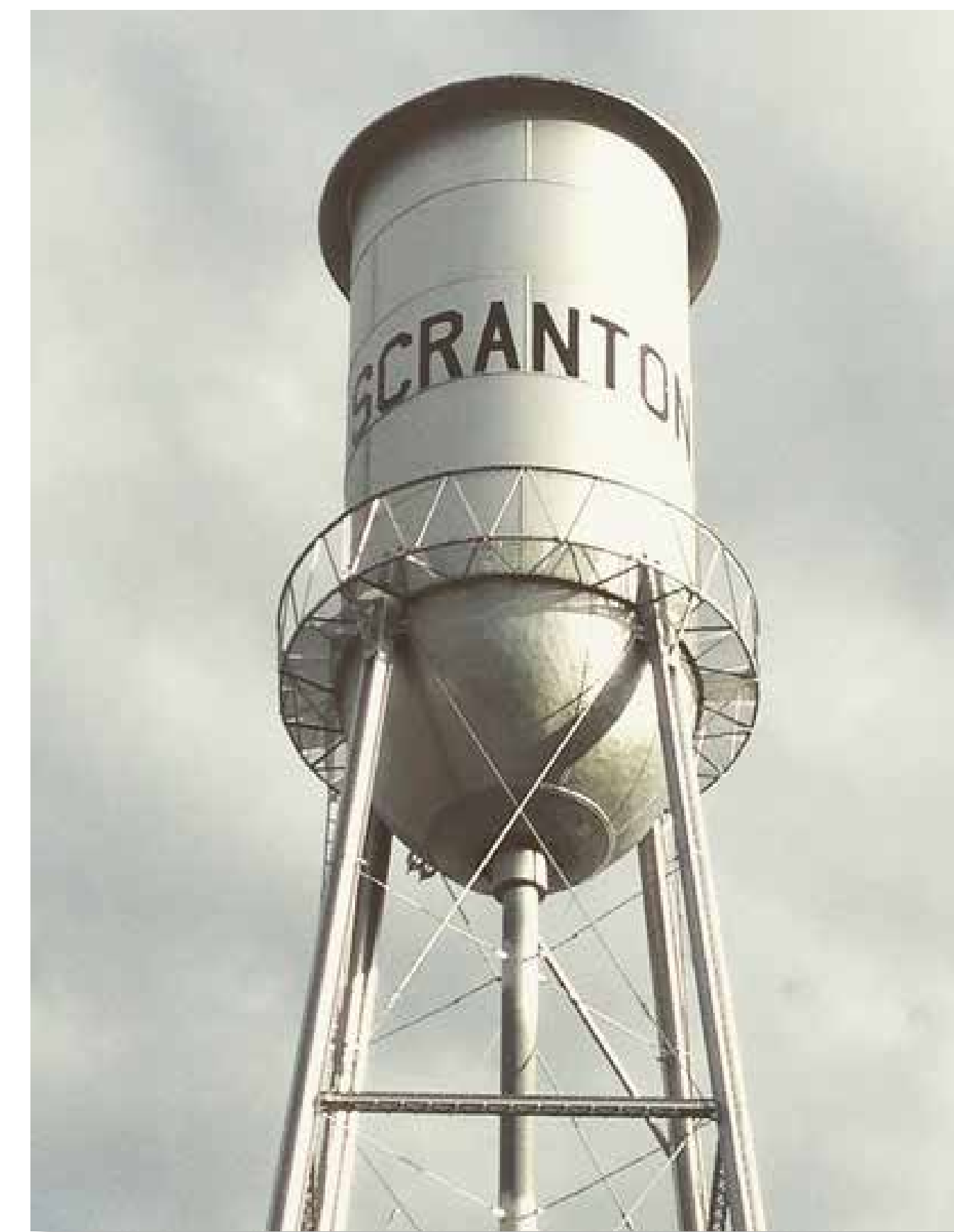
Scranton's water tower is the oldest working water tower in Iowa.
