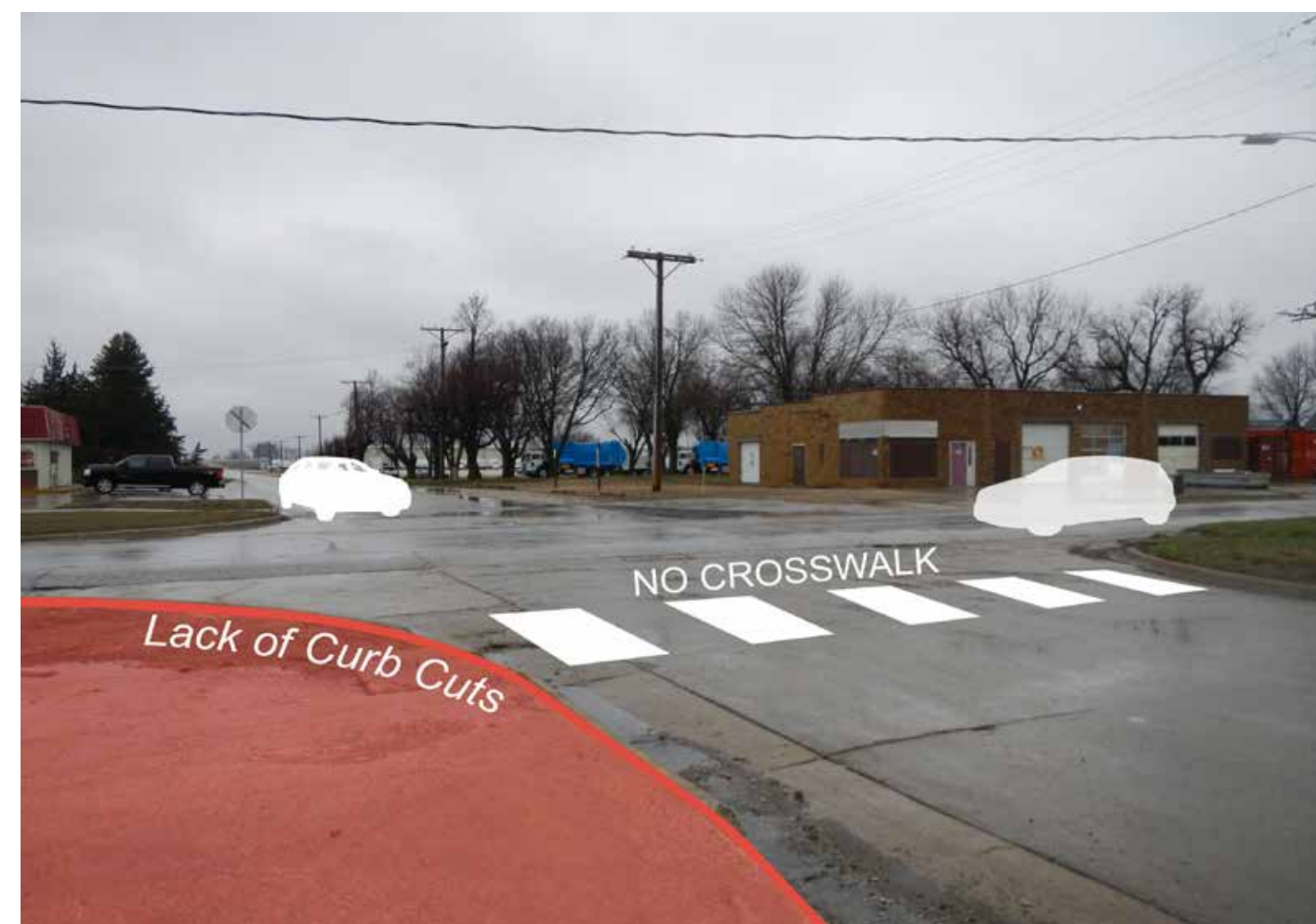
Barrier: Lack of Curb Cuts and Crosswalks at Hwy 25/State Street Intersection
