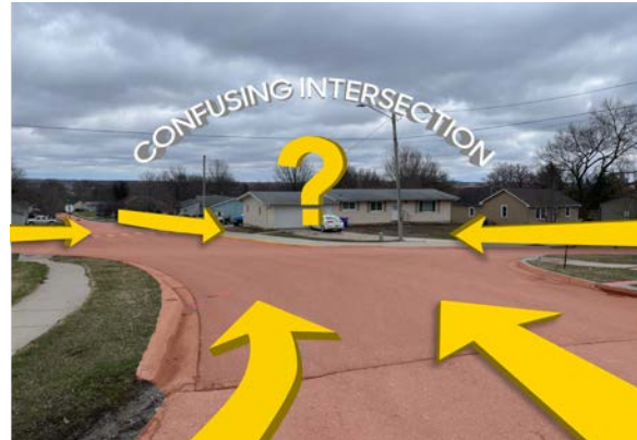
The five-way intersection of Ella, Elm, Blackberry, Palm and Ash Streets is disorienting for drivers, and it is difficult to see oncoming traffic.
