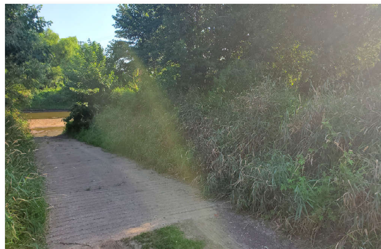
Existing boat ramp facing south from top of boat ramp
