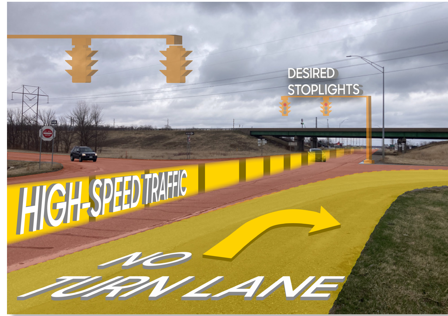
The intersection at Highways 22 and 218 is problematic and the site of multiple accidents due to lack of signage, no turn lanes, and high-speed traffic.
