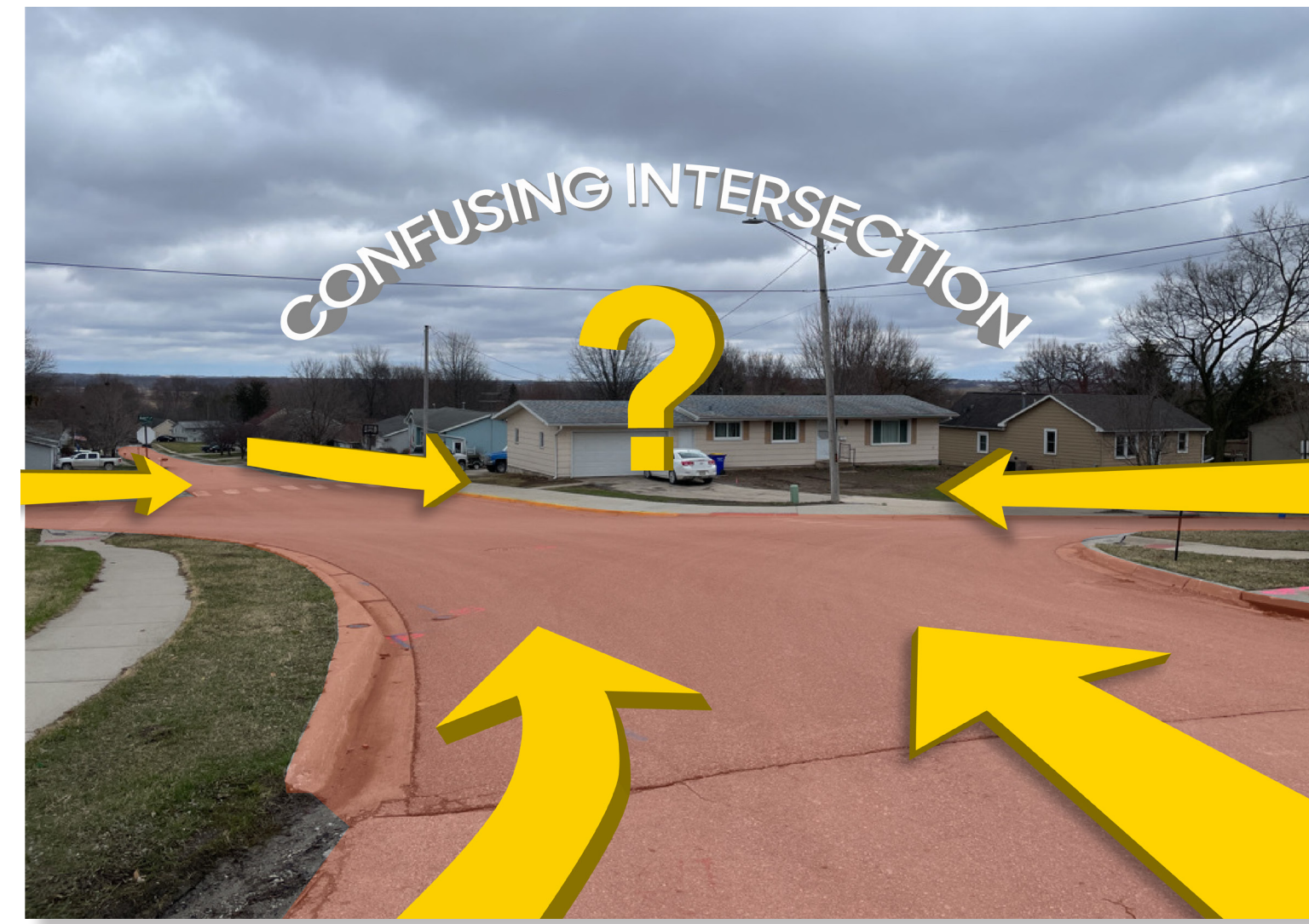
The five-way intersection of Ella, Elm, Blackberry, Palm and Ash Streets is disorienting for drivers, and it is difficult to see oncoming traffic.
