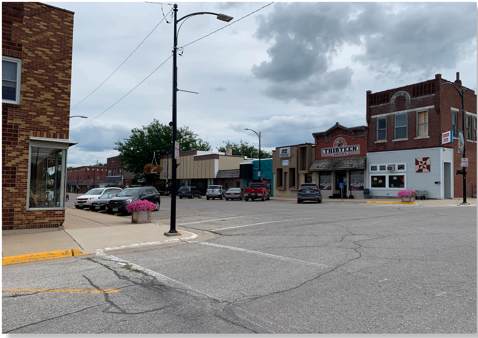
Existing conditions on the corner of Main Street and Blackhawk Street
