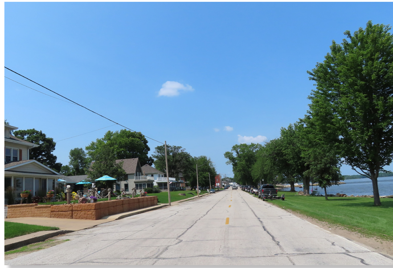
Existing: Photo taken along River Drive (just north of its intersection with Chestnut St.) and is looking northerly
