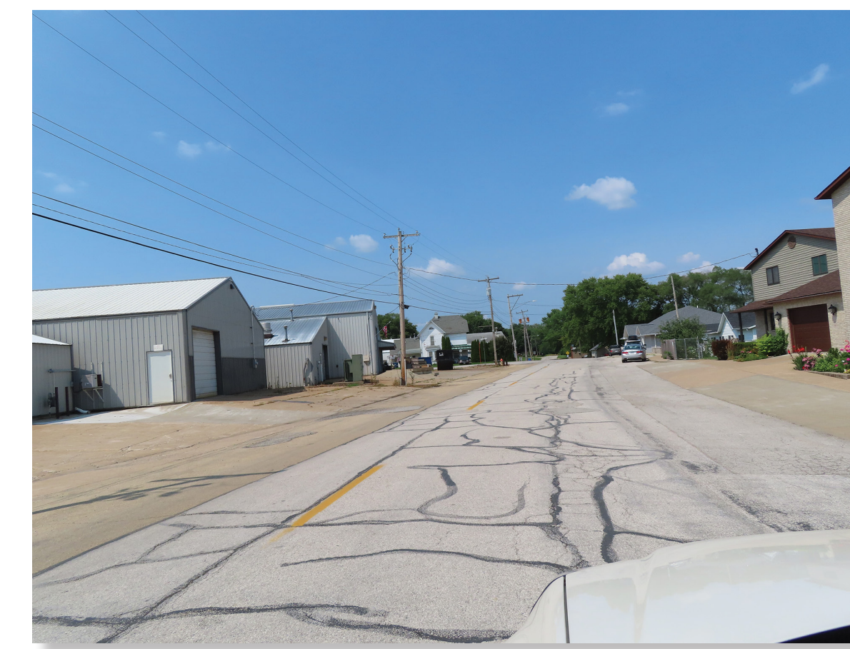
Existing: Photo taken at northern end of River Drive, just to the west of its intersection with Lost Grove Road and is looking northerly along River Drive
