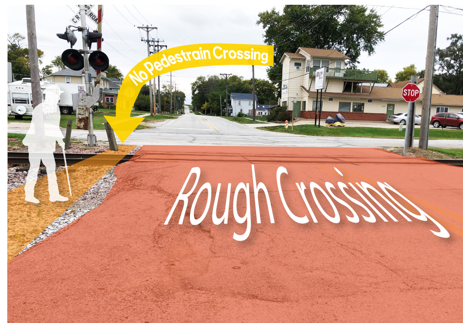
The railroad crossing on Lost Grove Road is difficult to cross because it is rough and there is no pedestrian crossing.
