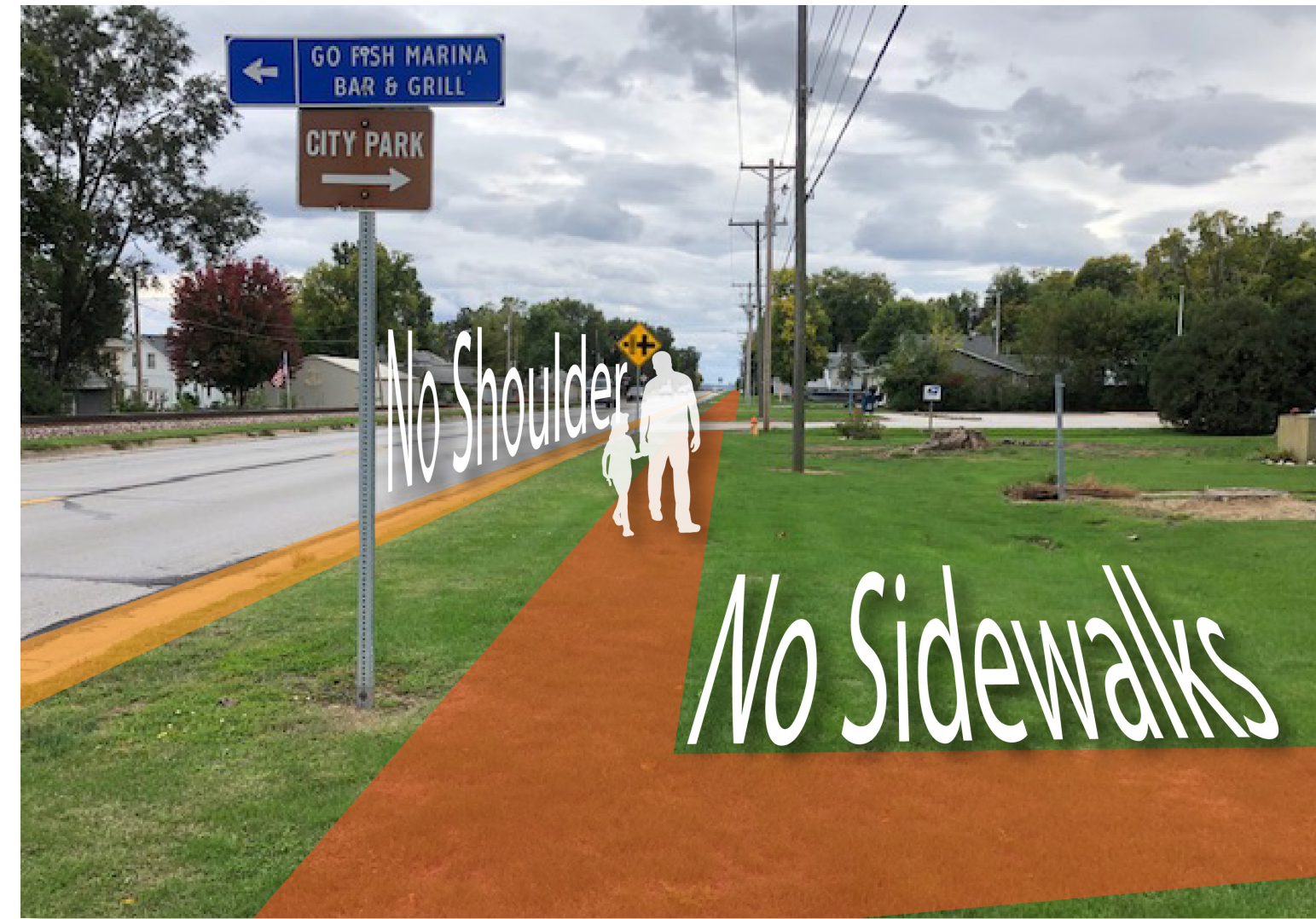
There are no sidewalks or shoulder on Highway 67, creating a barrier for pedestrians.
