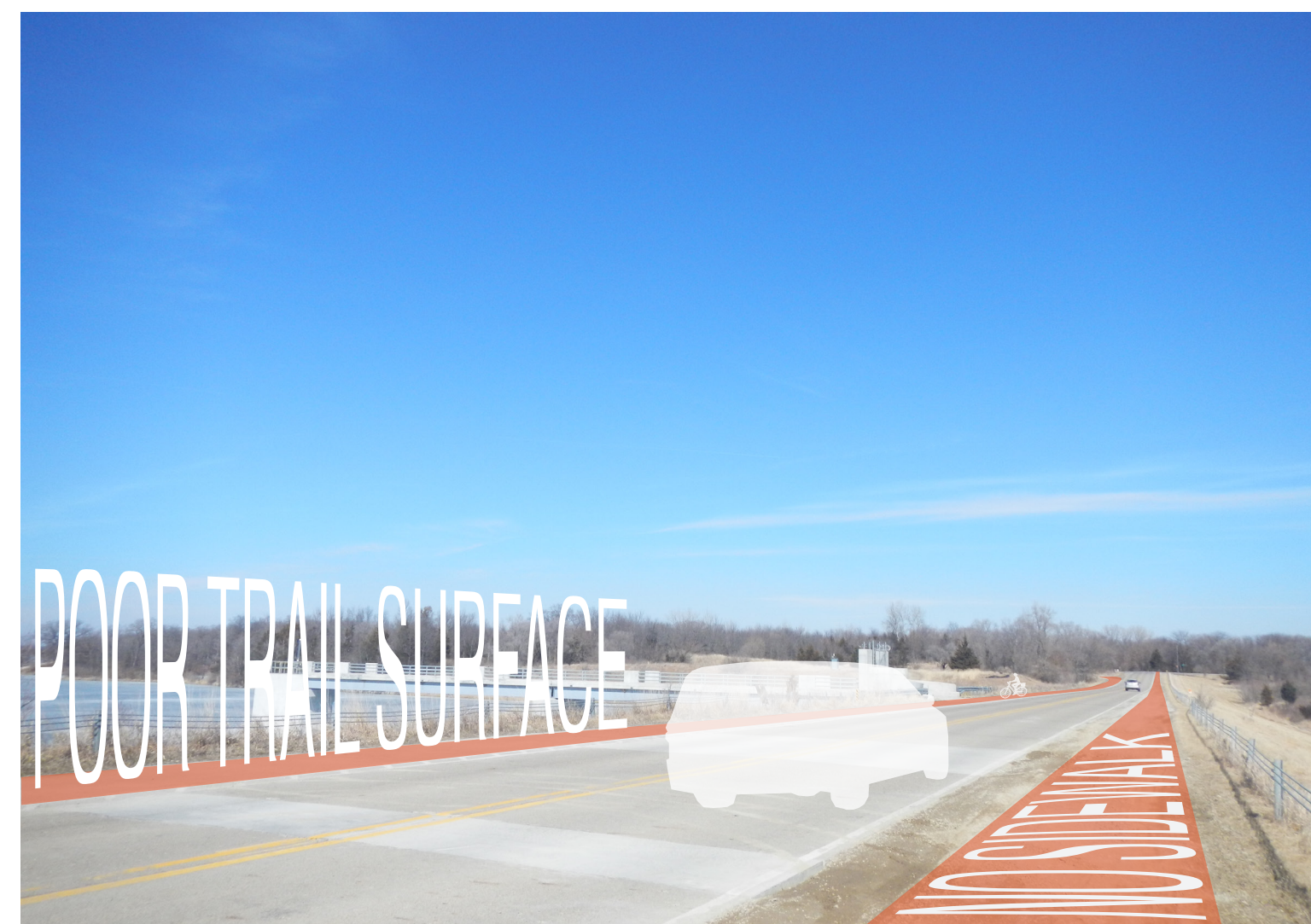
NW Big Creek Drive has no sidewalk (east side) or poor sidewalks (west side), effectively limiting access to Big Creek for pedestrians and cyclist.
