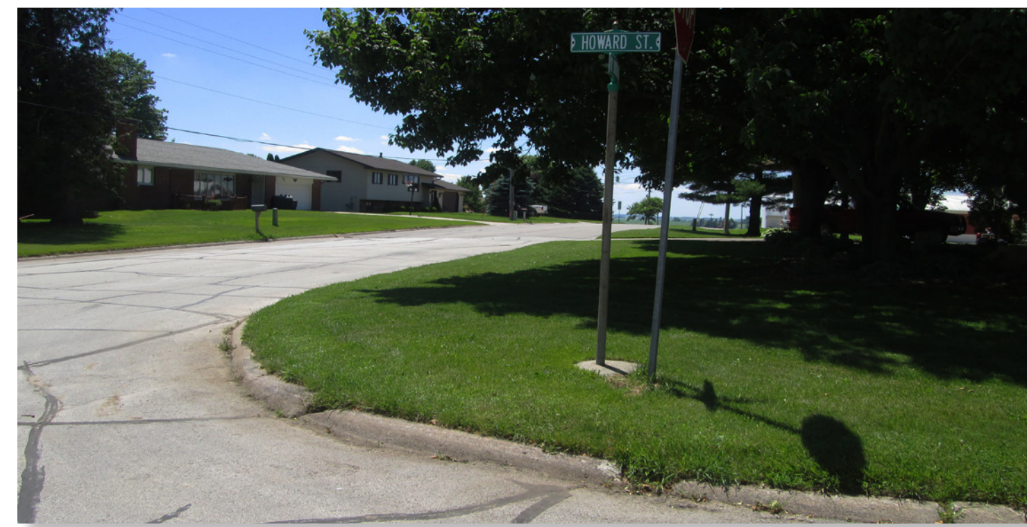
Existing sidewalk on Howard Street looking west.
