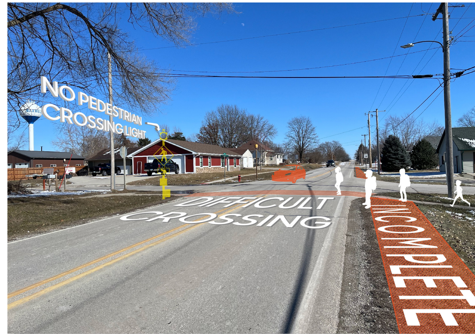
The sidewalks at the intersection of Metcalf and 5th Streets are disconnected. Speeding traffic on 5th Street makes it difficult to cross without a crossing light.
