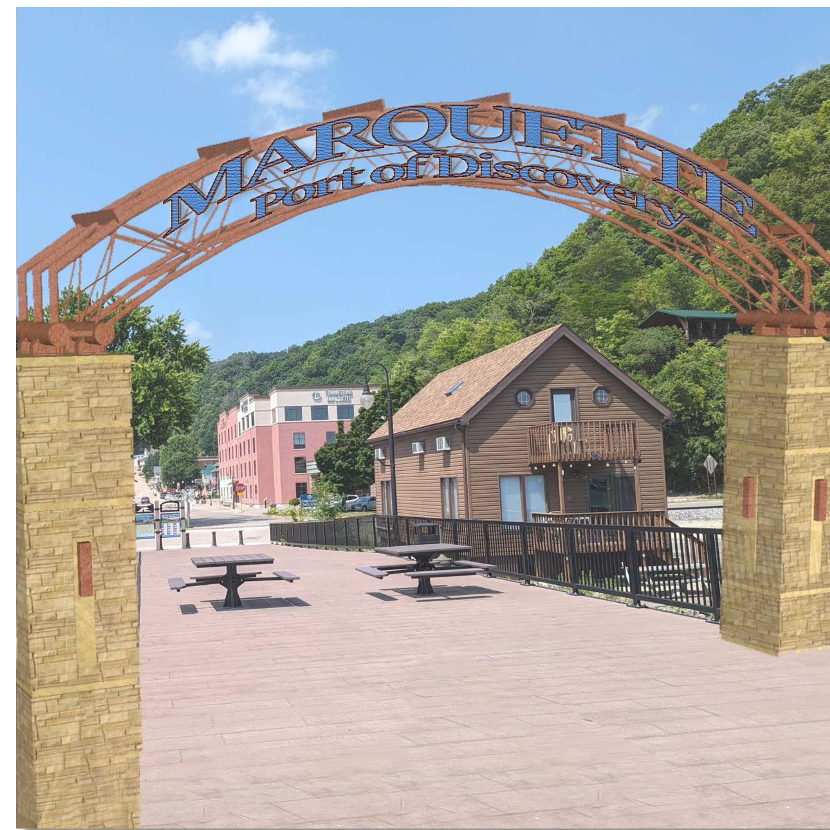
Entry archway for Marquette located on the pier at the Riverfront Boardwalk and Marina. Limestone columns flank each side of the pier and a Corten steel archway features lettering that will be illuminated at night.
