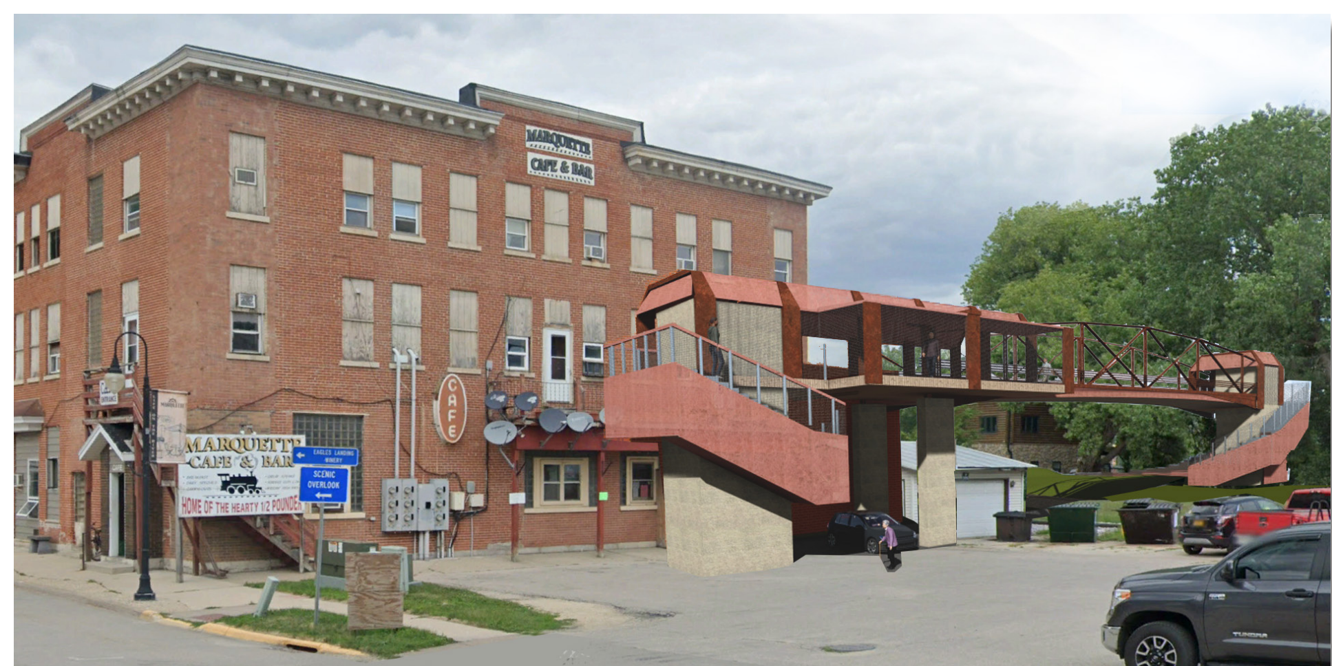
1.) The pedestrian bridge with elevators at Edgar Street crosses the railroad tracks, providing access between the Riverfront Marina and downtown. It will also connect to the second story of the adjacent building.
