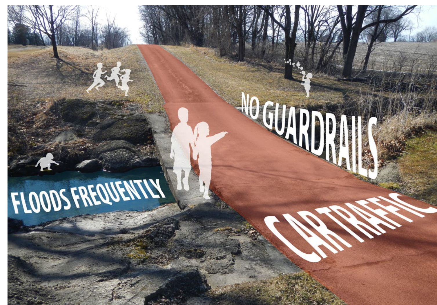
The bridge into the park is in need of repair and floods frequently, blocking access to the park entirely.
