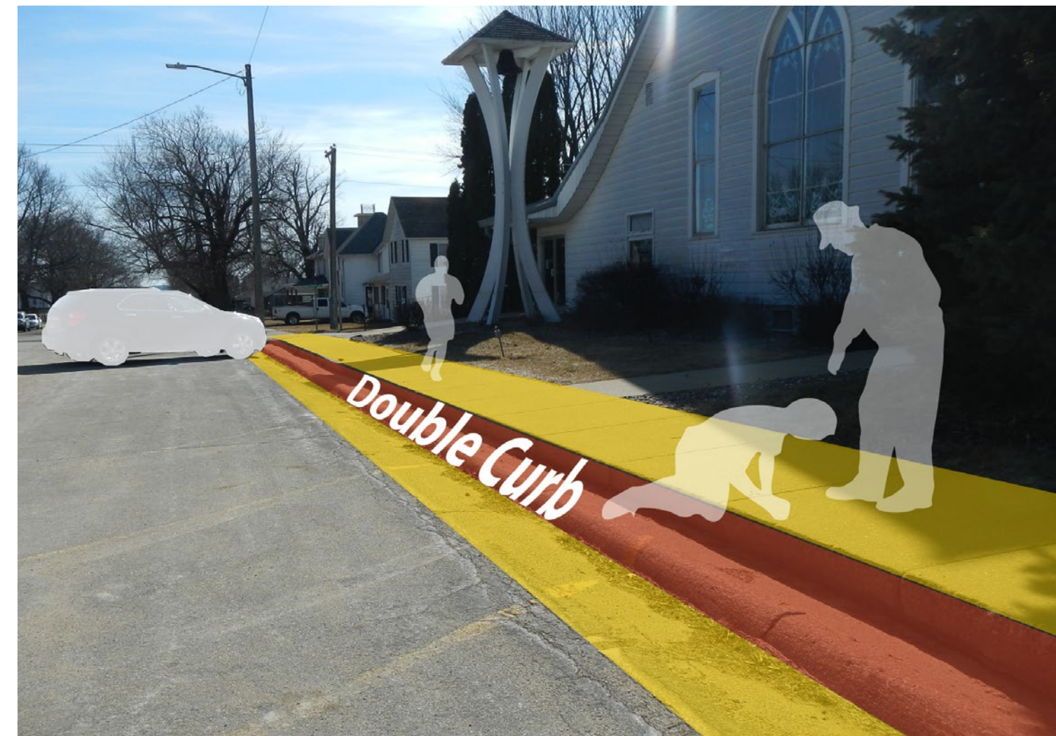
The double curb in front of the Presbyterian Church is a trip hazard especially during the winter, when it can be hidden by snow.
