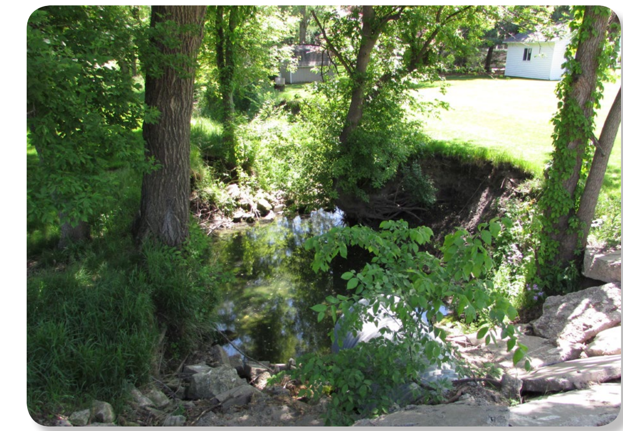
Streambank Near 11th Street and J Avenue
