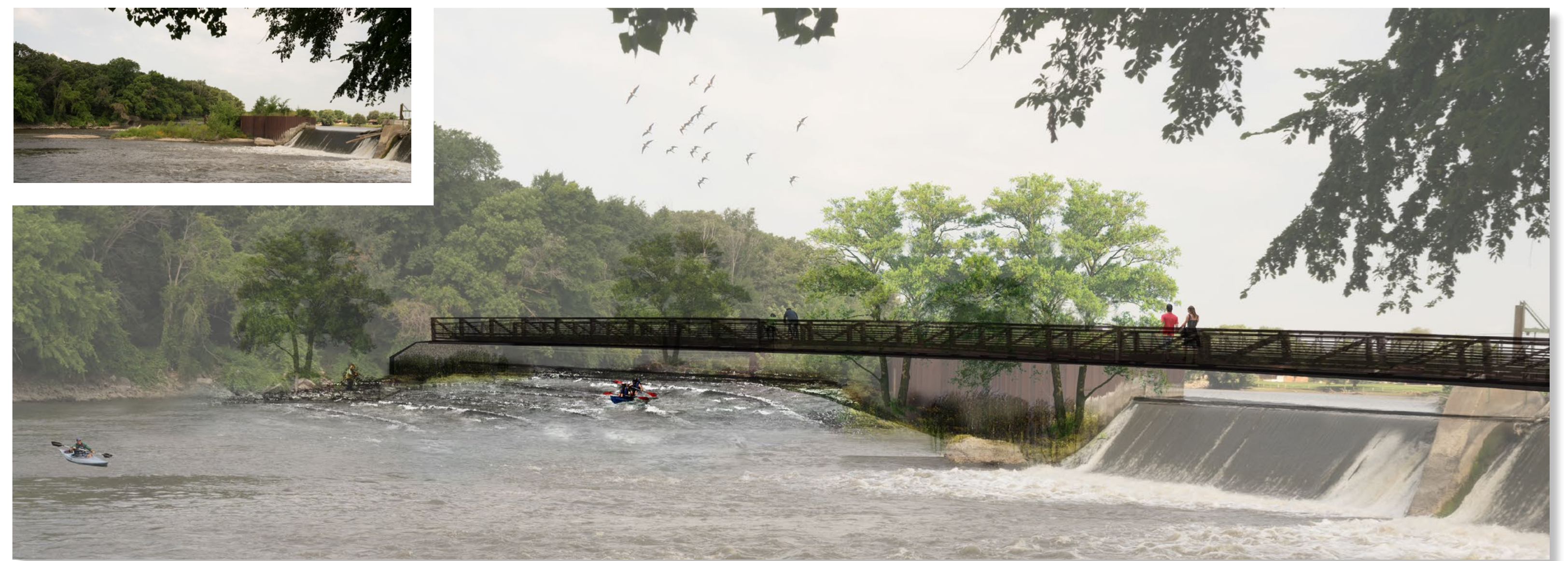
Option 1: Dam with One Side Altered (roped-off area on the upstream side to prevent boaters from going over dam)
