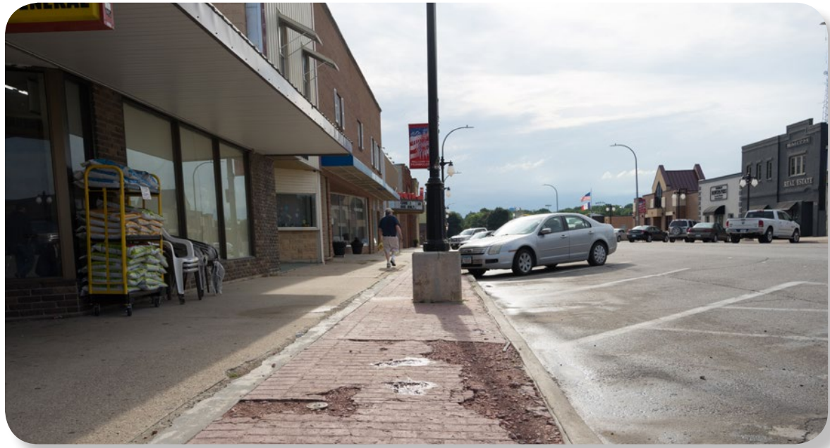
Existing sidewalk conditions on Sumner Avenue
