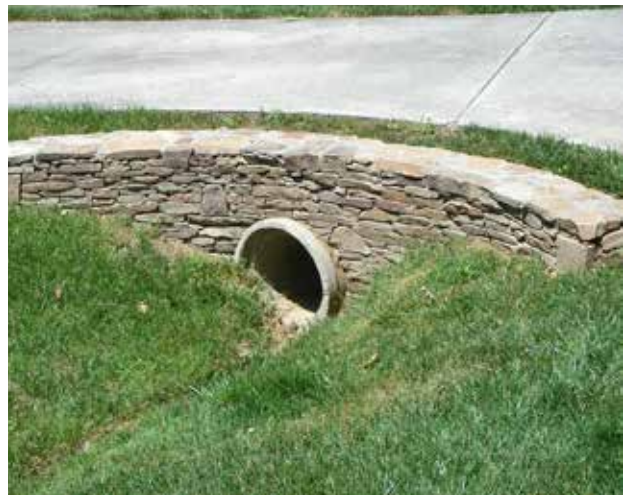
Pictured above: Example of a culvert inlet which would allow water to flow through existing Perrin Park trail dike in flood events
