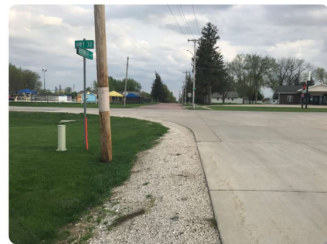
No Pedestrian Crossing at Highway 30 & Arizona
