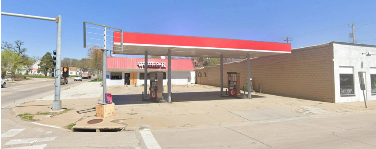
Existing | Corner of Locust and Sharp Streets
