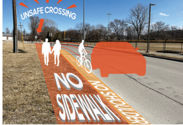
A lack of sidewalks, road shoulder, and marked crosswalks creates intimidating conditions for pedestrians and cyclists accessing Sivers Road.
