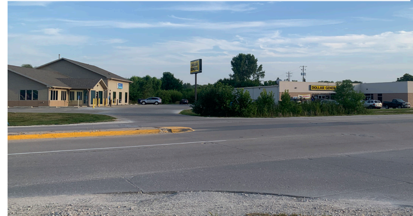
Existing Conditions | Locust Street
