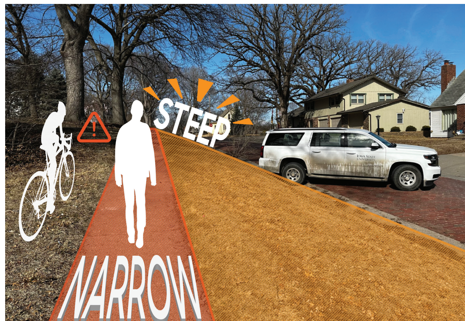
The steep incline from the road create challenges for some to access the sidewalks on Myrtle Street. Walkers and cyclists often go into adjacent yards when meeting someone on the sidewalk because it is too narrow.
