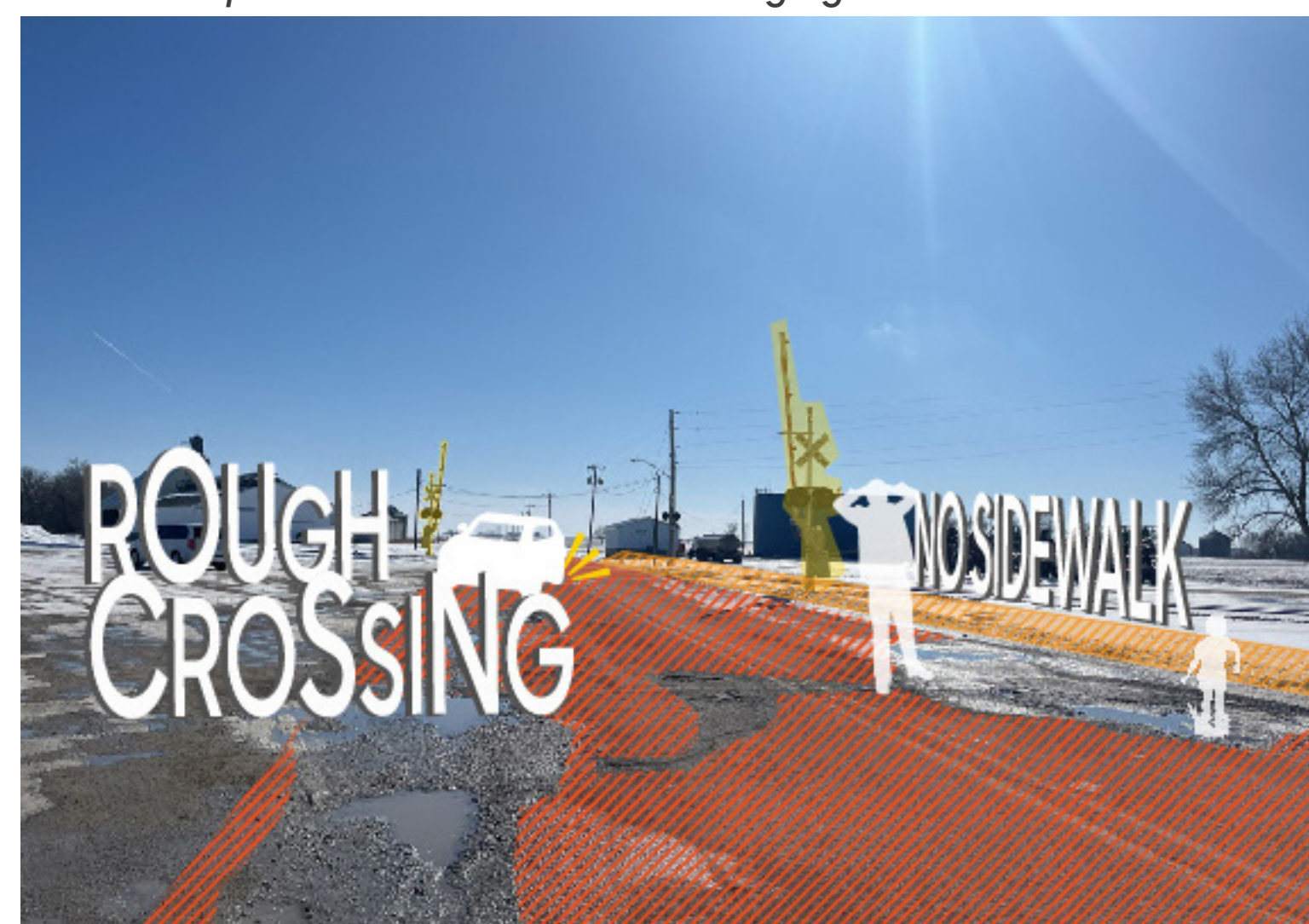
Dips in the roadway and degraded surface conditions make for a rough railroad crossing on Gilmore Street. Pedestrians do not have dedicated access along this route or for crossing the tracks.
