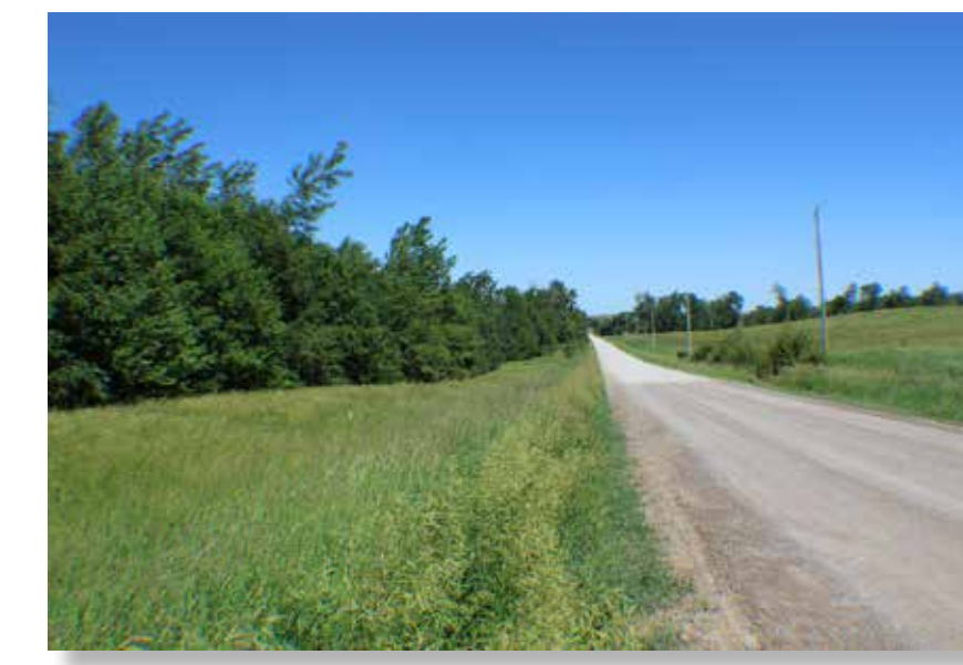
Existing conditions along 60th Street.
