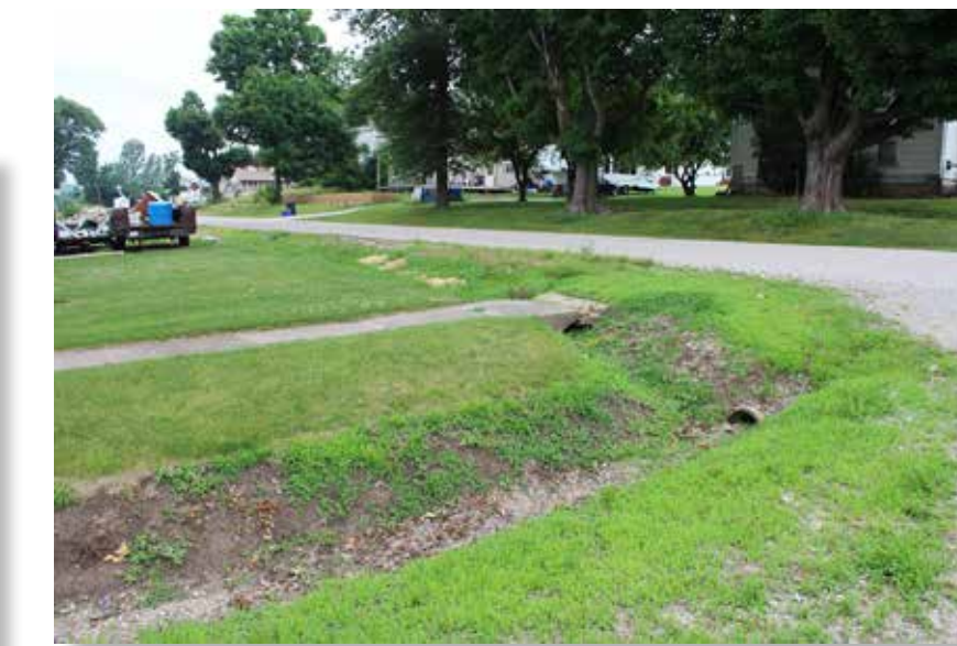
Existing conditions along E. Maple Street at Linden Avenue (SW corner).
